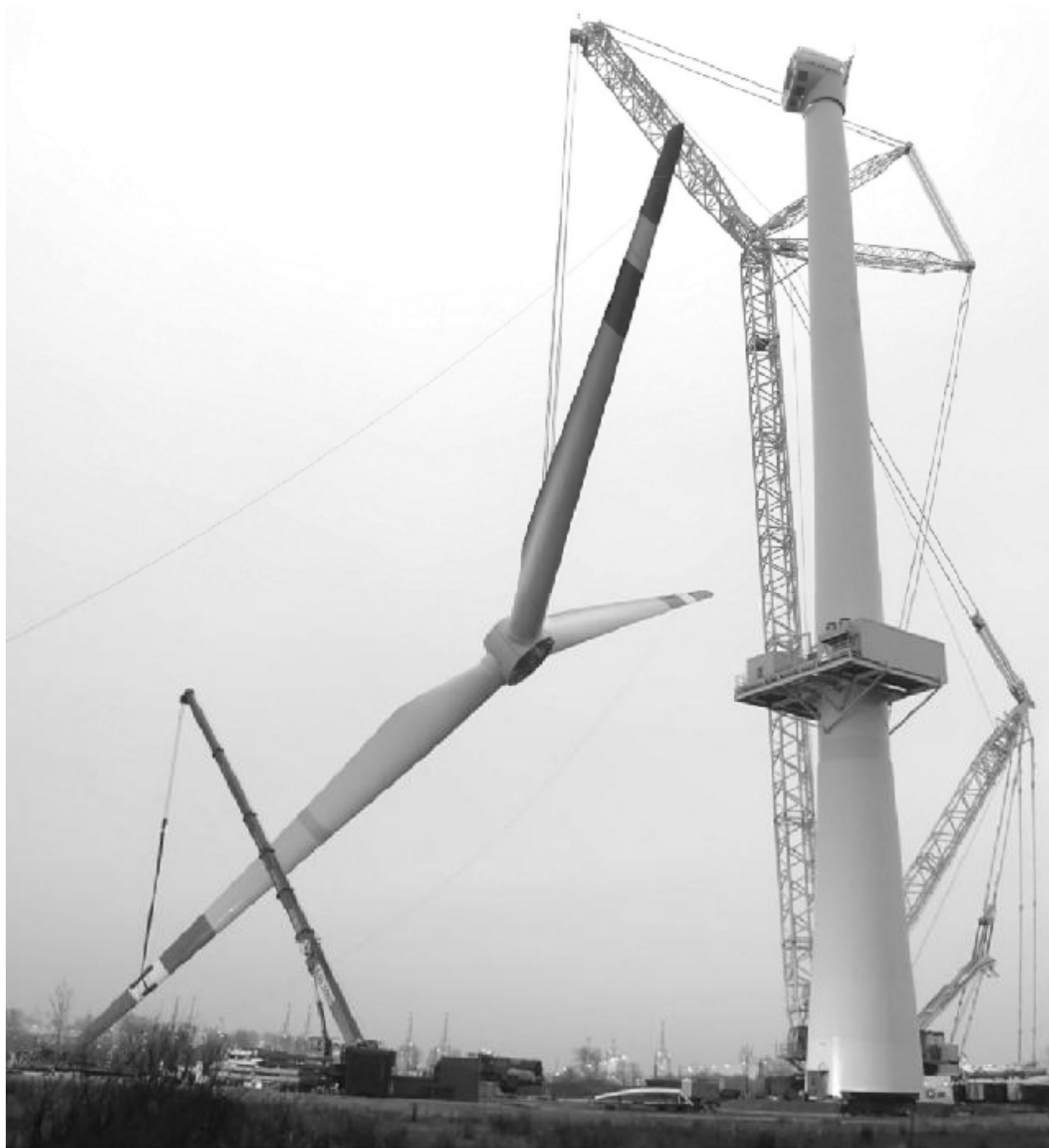
Fig. 15-13 Hoisting the Rotor by means of main mobile crane and assisting mobile crane [9]
